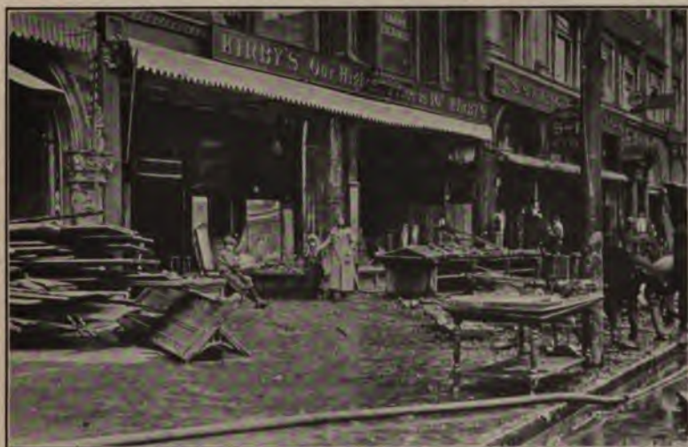
FIG. 2.—Cleaning up after the Dayton flood.
